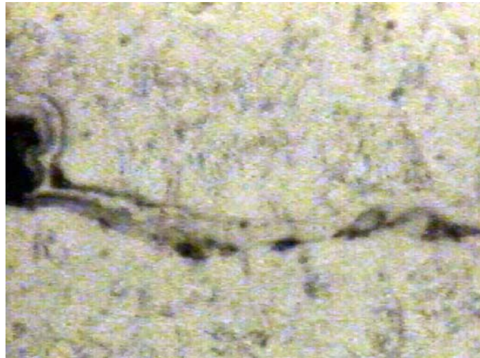
Figure 7 - Precursor - Inclusions that Coalesce into Cracks – Two Cracks Forming
